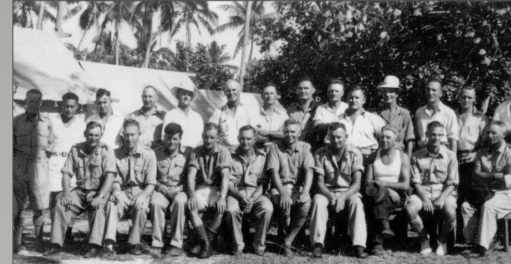
Airfield construction team from New Zealand Public Works (1942)
